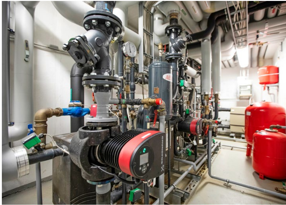
District heat is delivered to the heat distribution centre for processing. Yritys Helen provides an overview of its total consumption.
